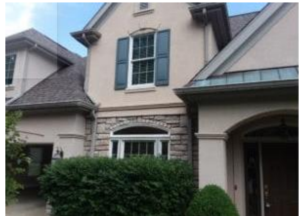
Figure 4. EIFS (Exterior Insulation and Finish System)
