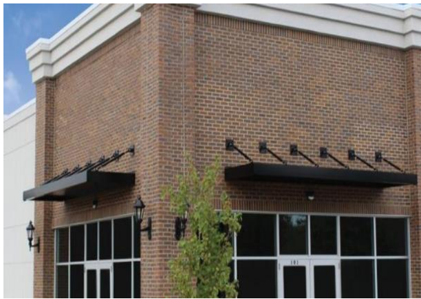
Figure 2. Masonry Veneer
