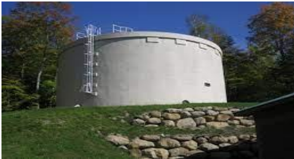
Figure 1. RCC water tank on earth's surface
