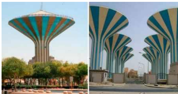
Figure 3. Elevated RCC Water Tank
