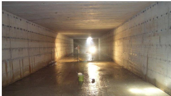
Figure 2. Underground Water Tank
